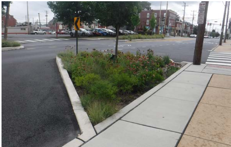
Figure 5.2-1. Typical Bioretention/Bioinfiltration System
