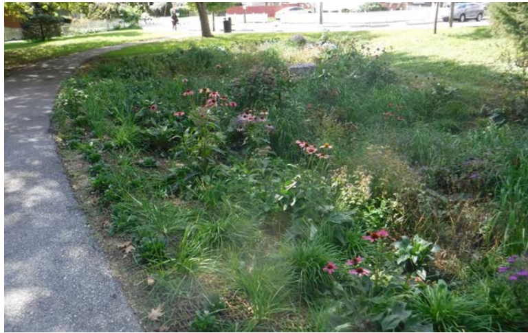
Figure 5.7.1. Typical Naturalized Basin System
