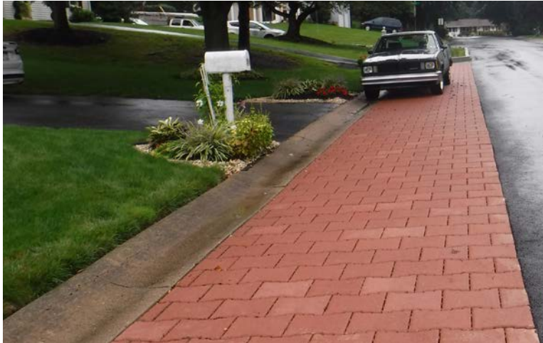
Figure 5.3-1. Typical Porous Pavement System
