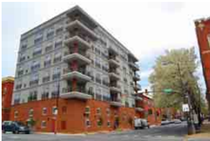
Recently completed Magnolia Place residences (Photo courtesy of LCA)
