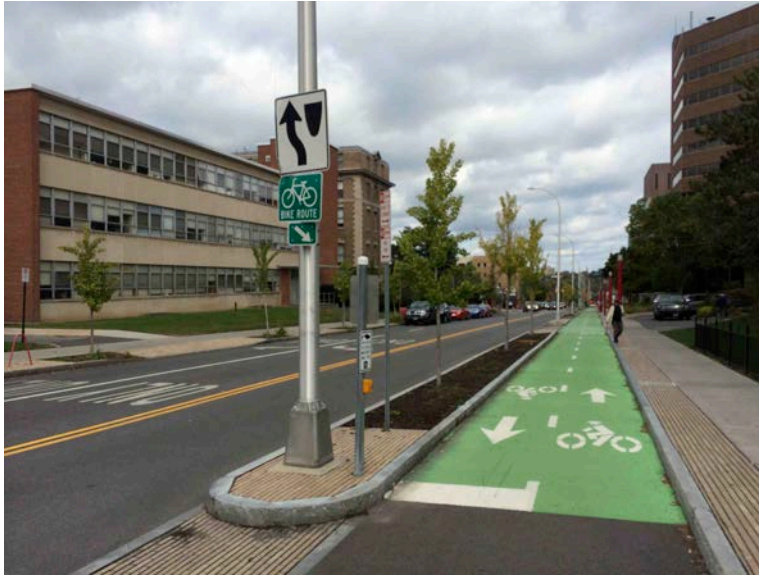
This methacrylate cycle track in Syracuse, NY, has held up well to weather.
