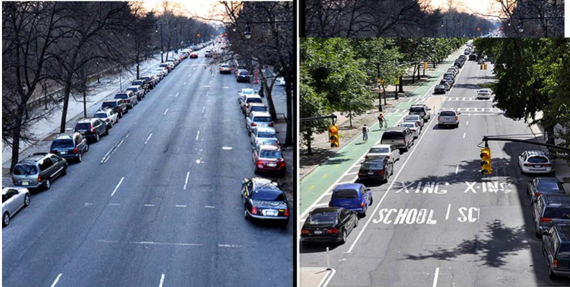
The insertion of a cycle track on this Brooklyn street dramatically improved safety for all road users without reducing daily car through-put.
