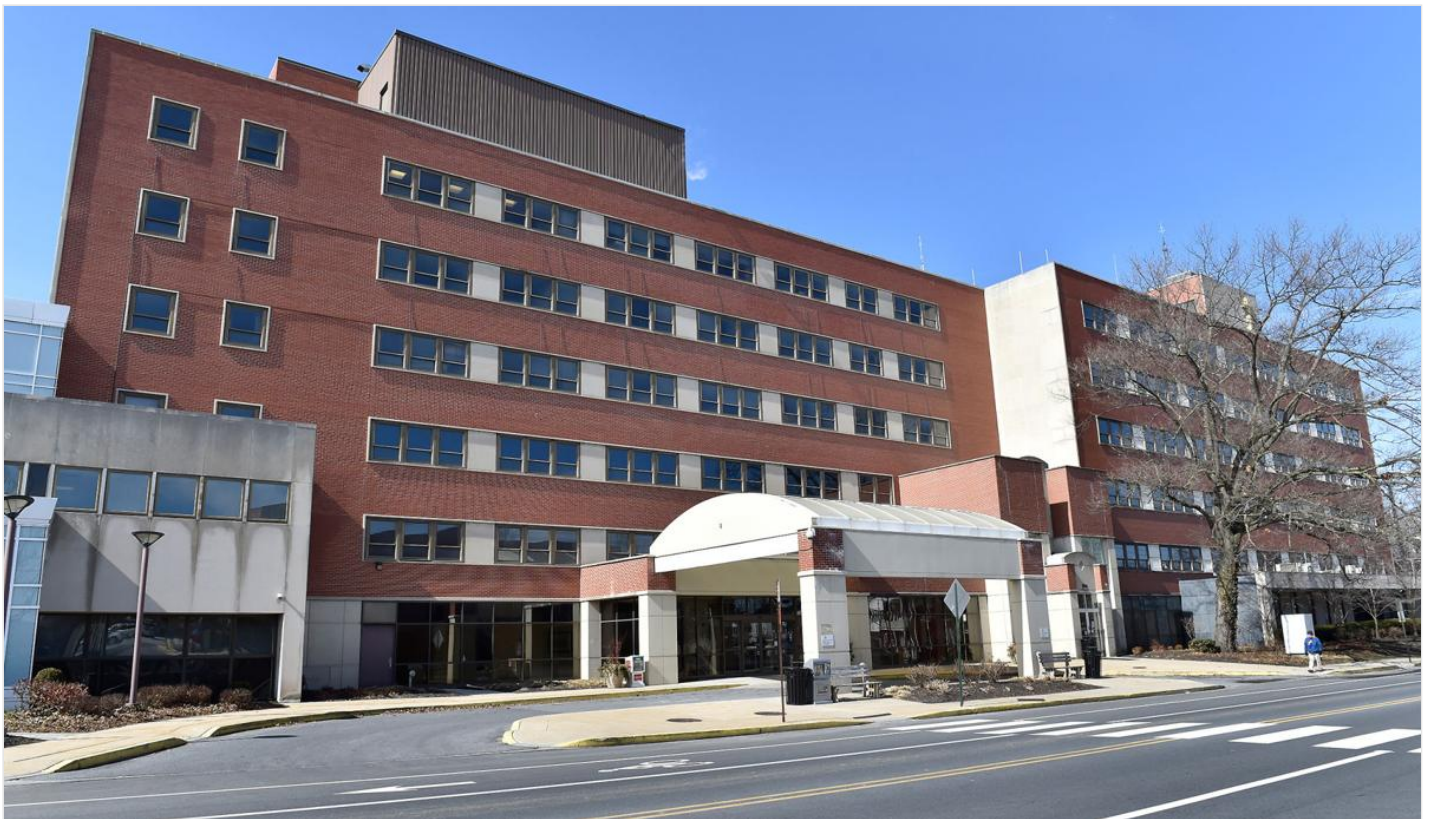
Homes, businesses could be in future for former St. Joseph's Hospital site
