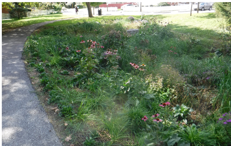
Figure 5.7.1. Typical Naturalized Basin System
