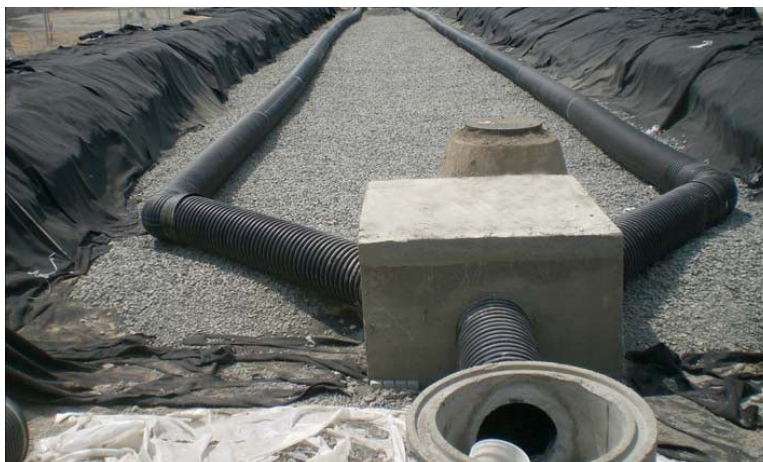
Figure 5.5-1. Typical Subsurface Infiltration and Detention System
