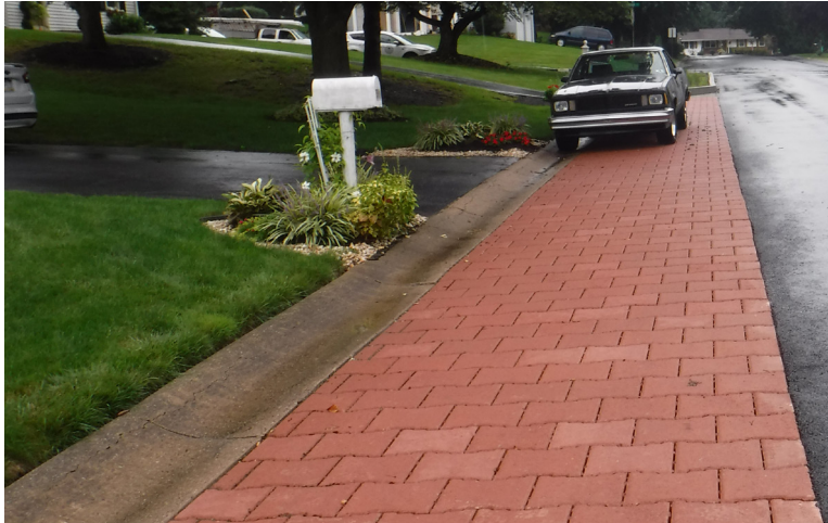
Figure 5.3-1. Typical Porous Pavement System
