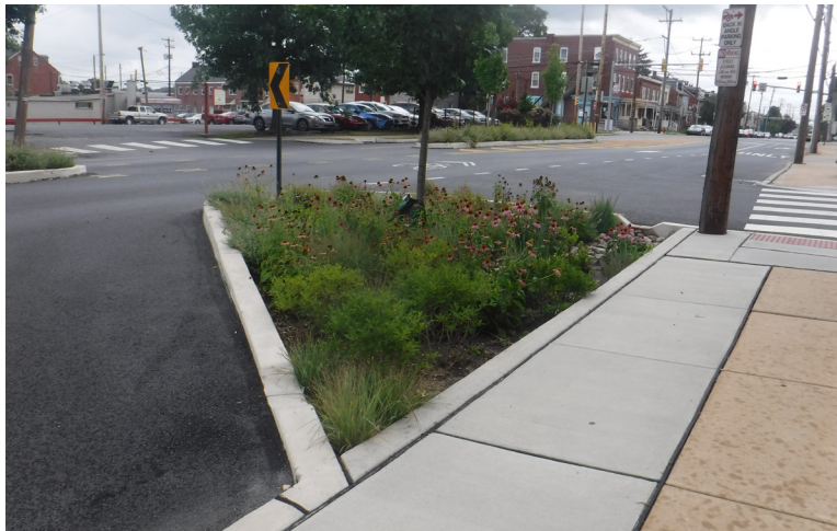
Figure 5.2-1. Typical Bioretention/Bioinfiltration System
