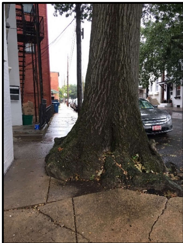
Figure 1-11. Sidewalk damaged by street tree
