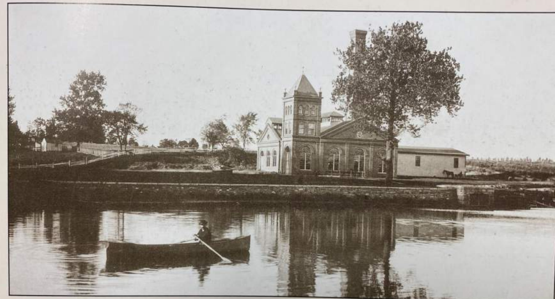
Lancaster Water Works, along the Conestoga River, circa 1892. The first Water Works operated on a combination of water power with an auxiliary steam power. This plant, built in 1888, operated solely on steam power. See photo below, where it appears in the background behind the Walnut Street bridge. Water was pumped from the Conestoga to reservoirs next to the County Prison on the ground now occupied by Reservoir Park.
