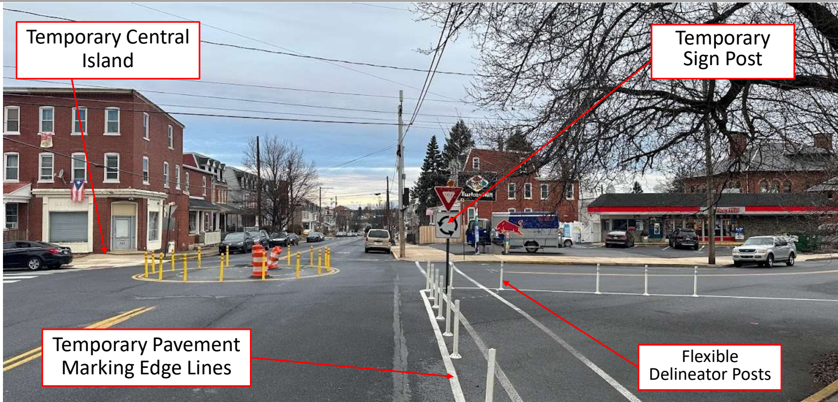
Elements of the temporary mini-roundabout installed in 2019
