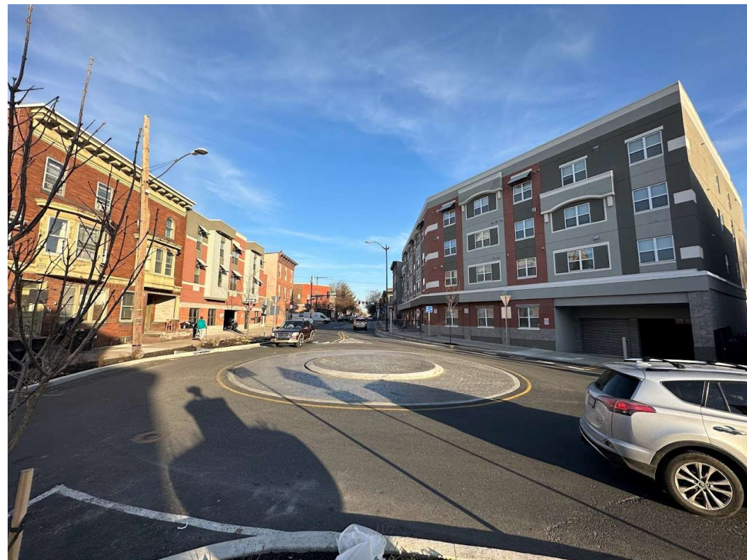
Mini-roundabout in Harrisburg, PA
