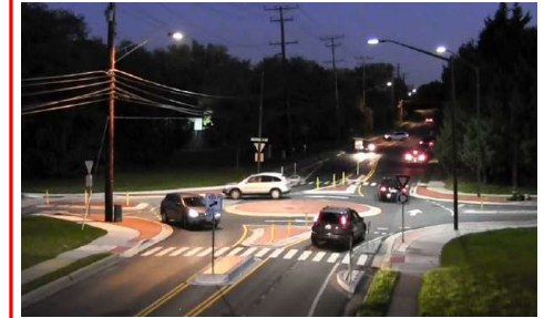
Street Lighting Enhancements + Signage
