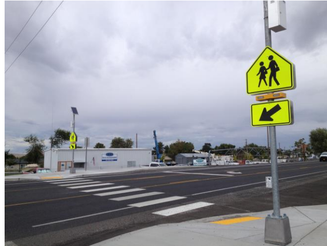
Rectangular Rapid Flashing Beacon
