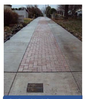
Alley 148 was redesigned to feature porous pavers atop an aggregate (gravel) infiltration trench.
