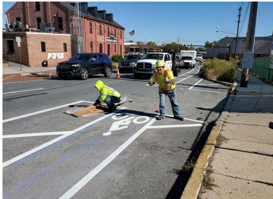
Walnut Street Repainting
