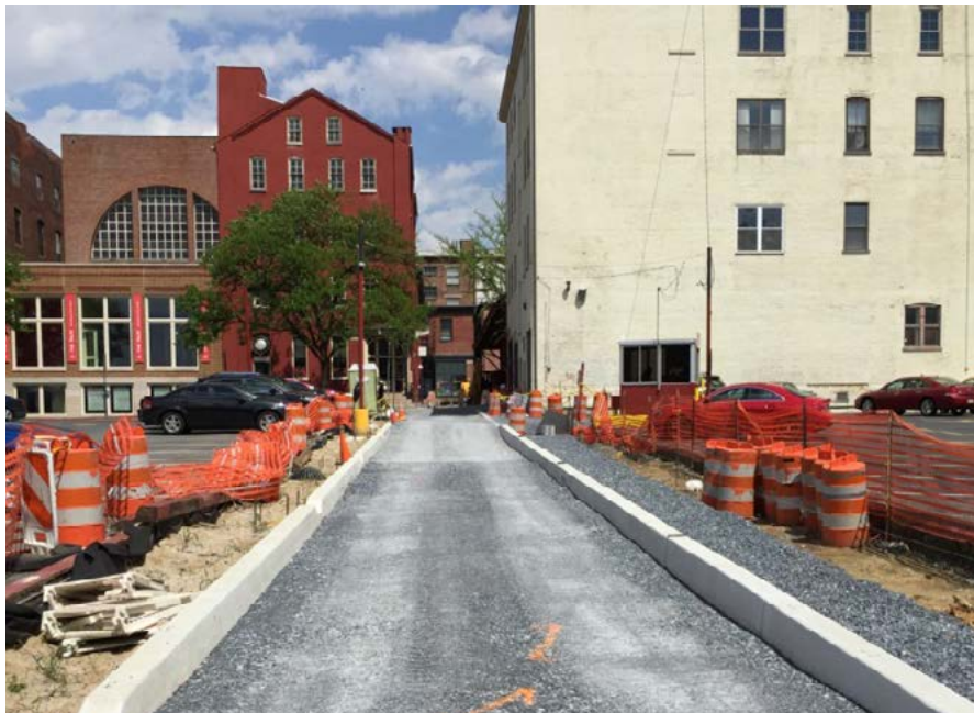
Grant Street Reconstruction
