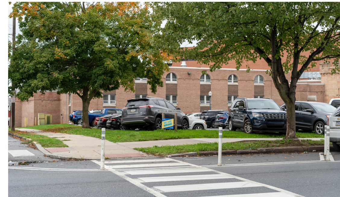
Daylighting resulted from Vision Zero plan can be seen on intersections along E King St. Photo Source: WRT
